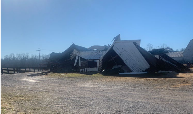
Damage to one of the barns at the UKREC beef unit
