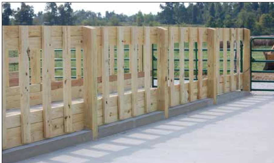
Figure 4-14. The vertical slats, of the winter feeding structure, provide containment of the conserved forage, which reduces waste by cattle. The raised feed table provides feed within reach of cattle, while limiting exposure to animal manure. A broomed concrete finish provides traction for cattle and vehicular traffic. The concrete surface also eases mechanical cleaning. (Metal feed panels can also be used as a substitute for wood).
