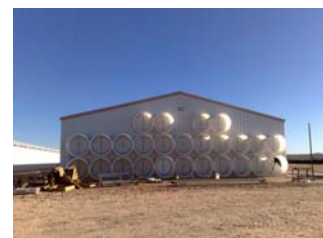
Figure 4 - Building with many tunnel ventilation fans
