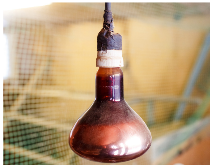
Figure 5. Heat lamp incorrectly used – a fire hazard
